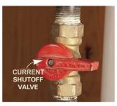
A new gas shutoff valve may need to be replaced if it is not up to code.
